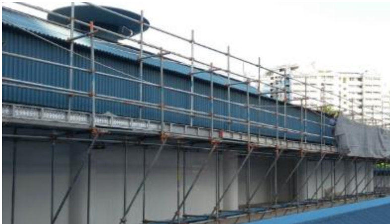
Figure 31 Cantilever Scaffold
