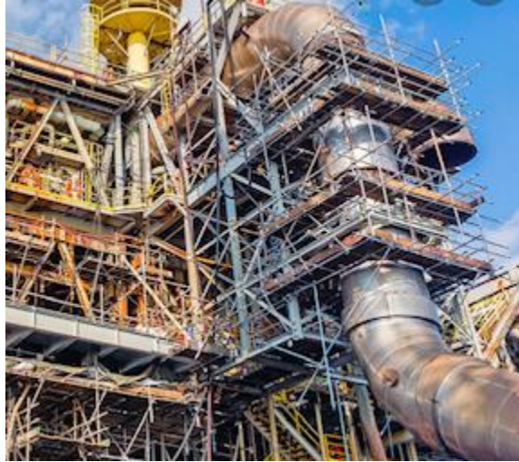
Figure 32 Tube and Coupler Scaffold
